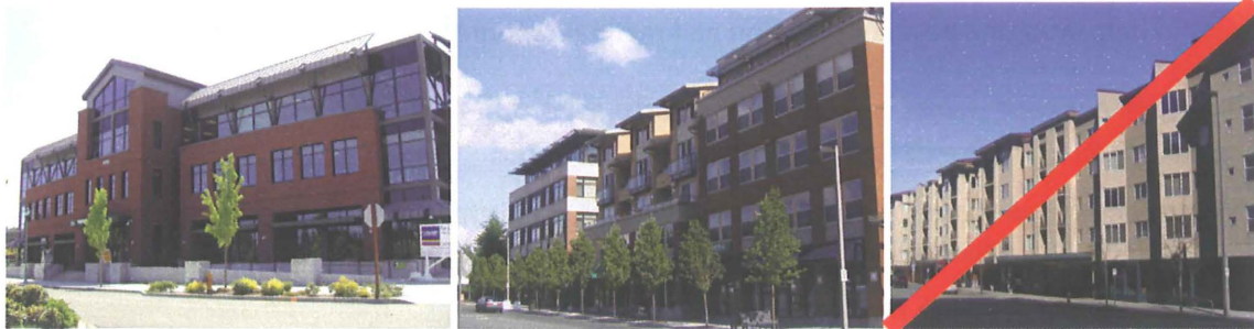
Figure 7 – Left and center images use substantial façade modulation and articulation; repetitive small-scale articulation in the right image does not successfully reduce perceived building bulk.
