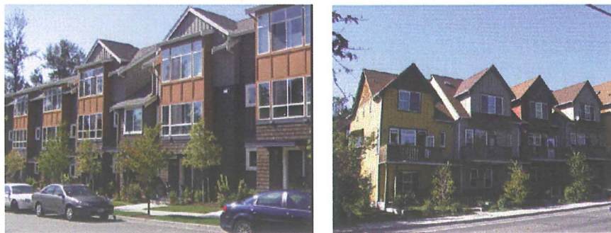
Figure 10– Appropriate multifamily and mixed use buildings that incorporate desirable design elements including canopies, decks, upper level setbacks, trellises and varied roof forms.
