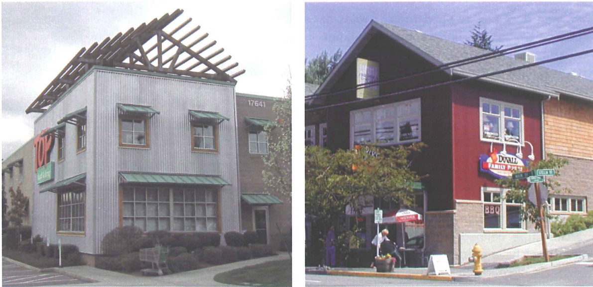
Figure 11 – Desirable architectural character using appropriate materials and emphasize window and corner elements properly.
