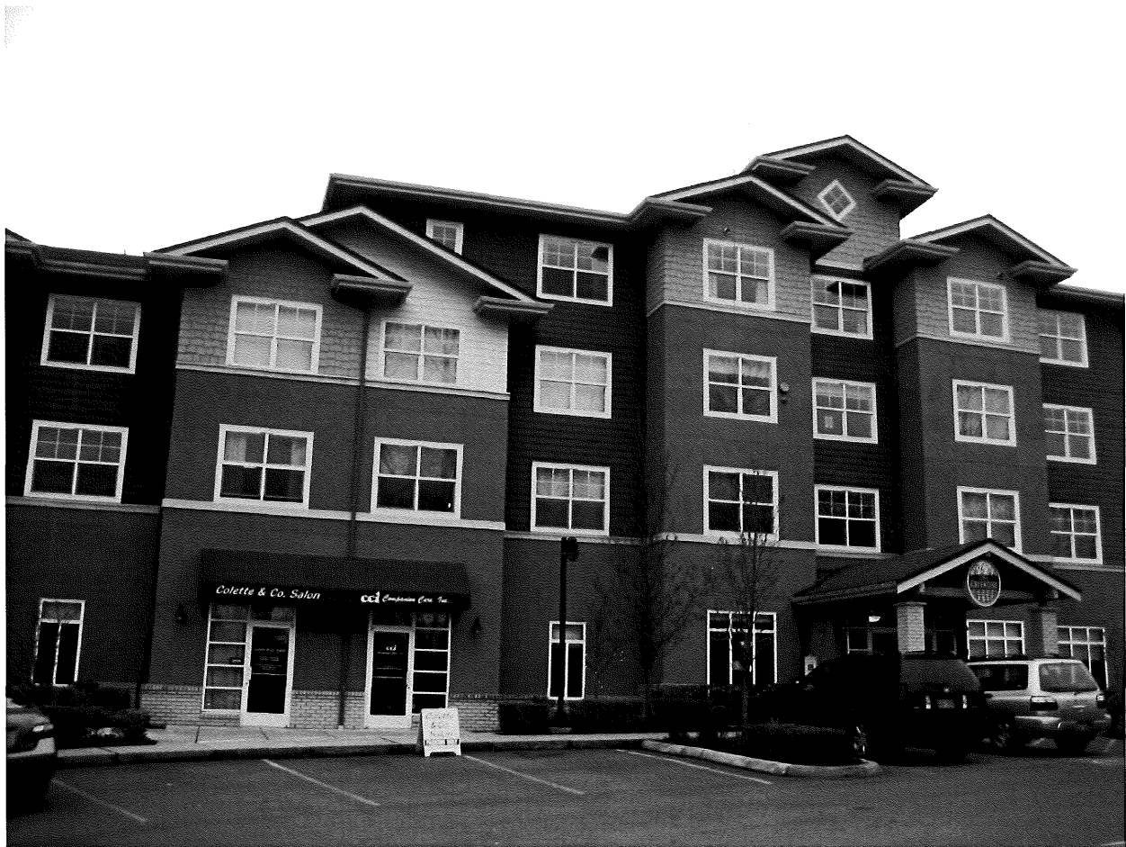
Figure 19 – Mixed-use building that shows variation in siding material
