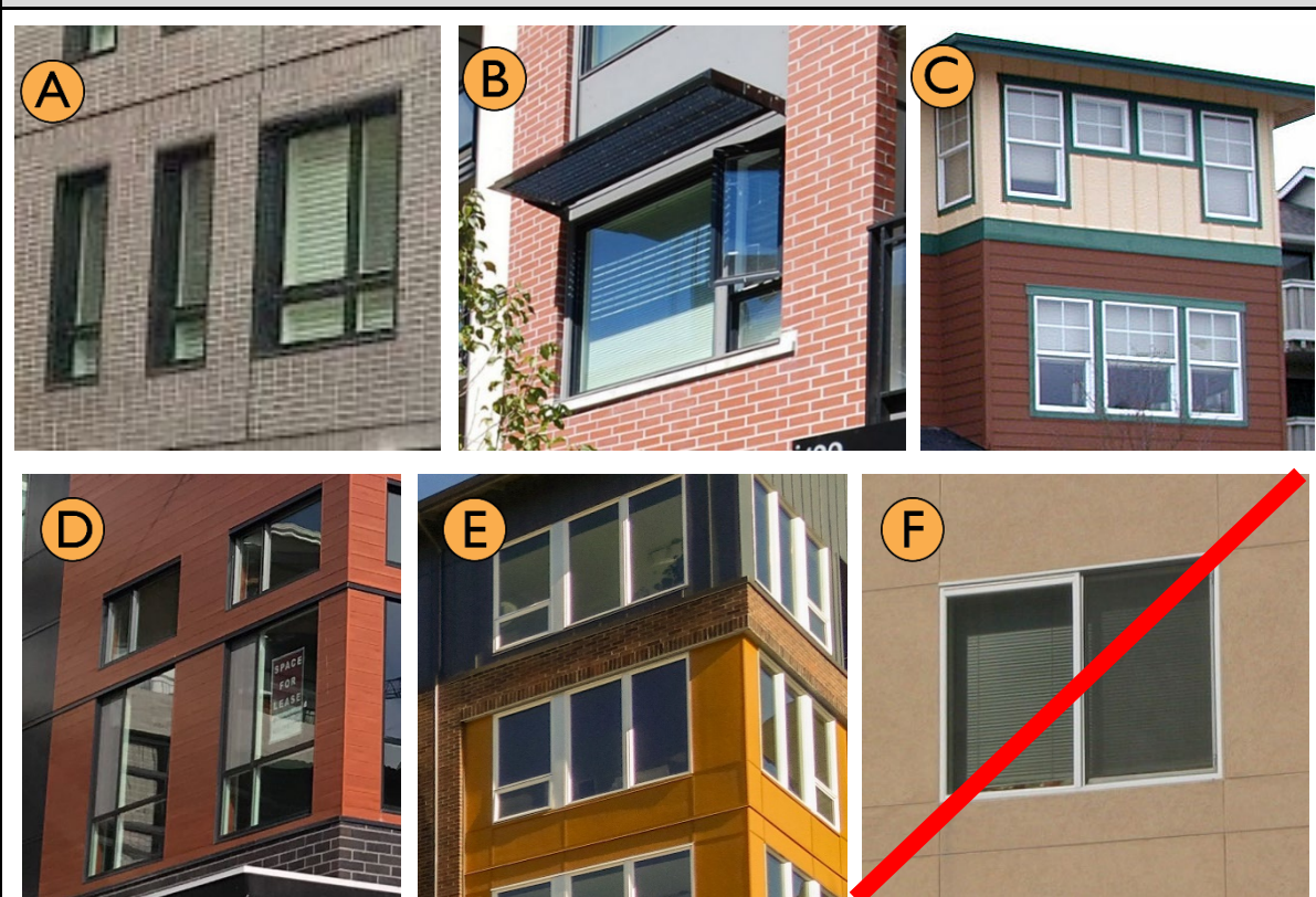
Figure 15. Acceptable and unacceptable window design examples.
