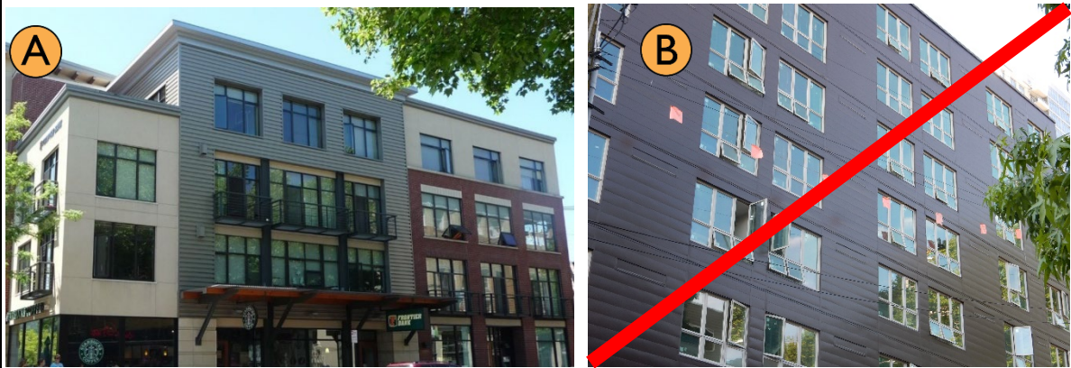
Figure 18. Acceptable sheet material siding examples.
