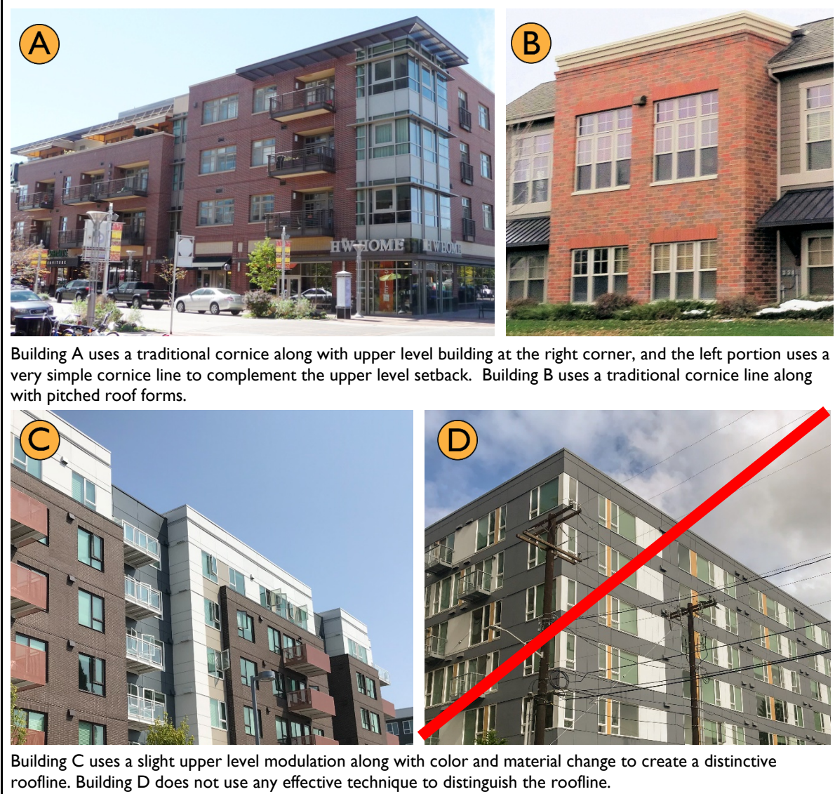
Figure 16. Examples of buildings employing a distinctive roofline that effectively provides an identifiable “top” to the building.
