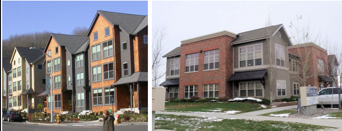
The left building illustrates a pitched roof example and the right building includes a combination of flat and gabled rooflines.
