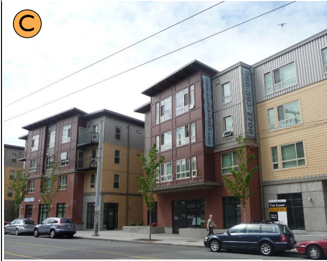
Figure 18. Acceptable sheet material siding examples.
