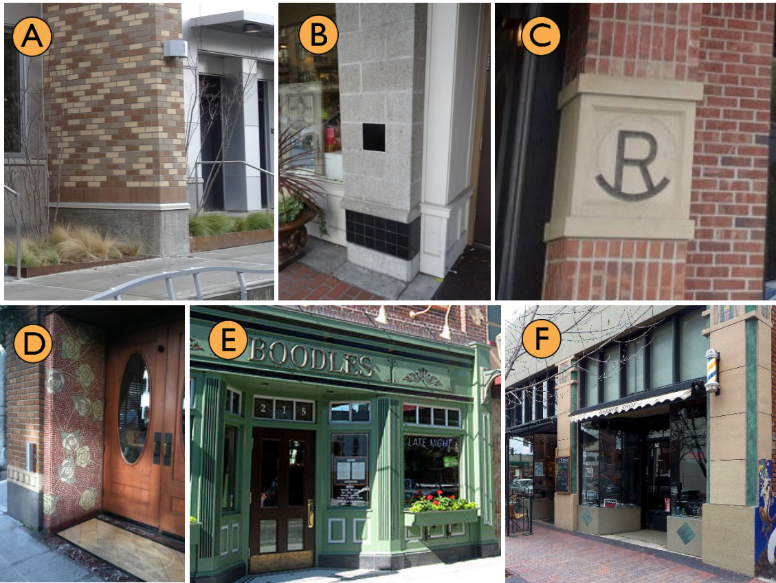
Examples of decorative surface materials. A = decorative brick/design. B = decorative tile-work and column pattern. C = decorative medallion. D = decorative mosaic tile work. E = decorative bulkhead. F = decorative tile-work and column pattern.
