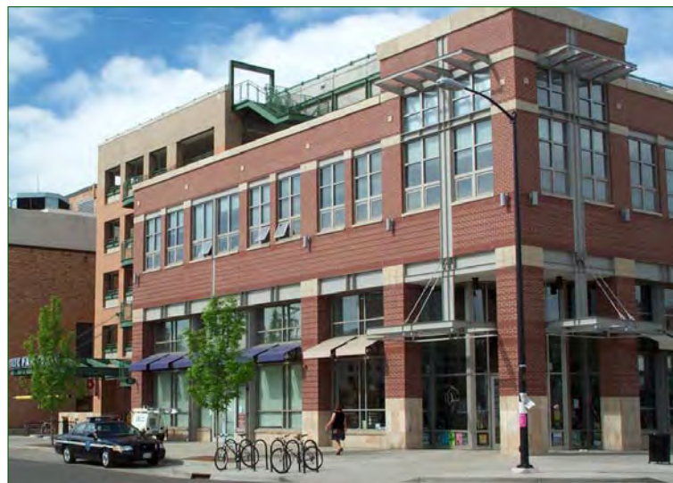
This parking structure incorporates a wrap of retail stores along the street edge. The storefronts are contemporary interpretations of the historic downtown context. (Boulder, CO)
