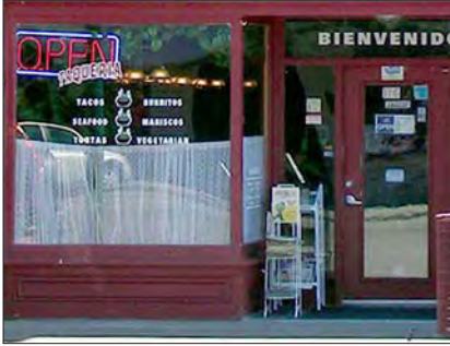
The kickplate pictured beneath this display window includes appropriate historic details.
