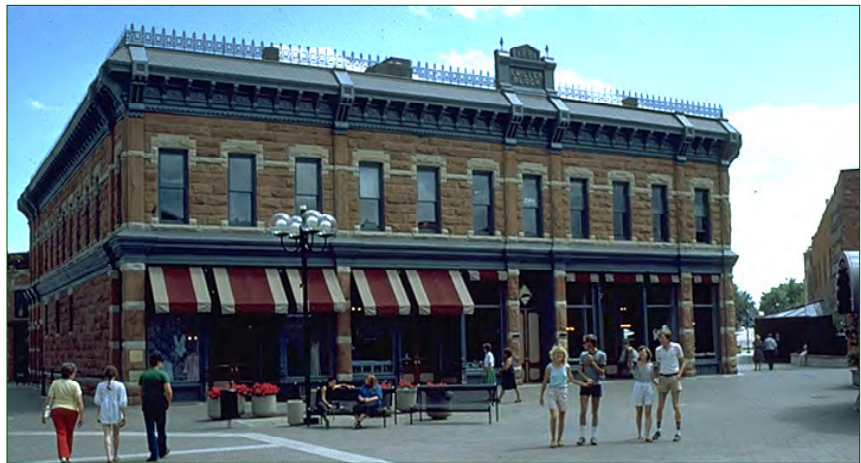
Storefront windows are reopened and upper-story windows are repaired. (Fort Collins, CO)
