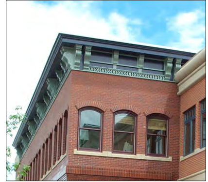
This image illustrates a modern interpretation of a traditional cornice. (Boulder, CO)
