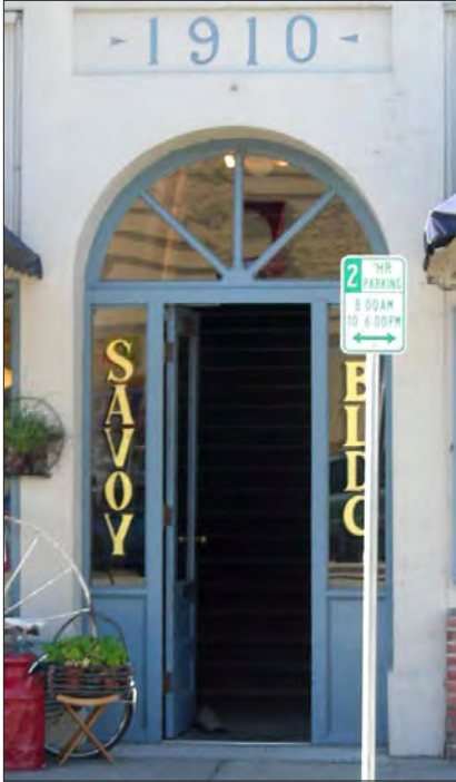
Historic doors are character-defining features and should be preserved.
