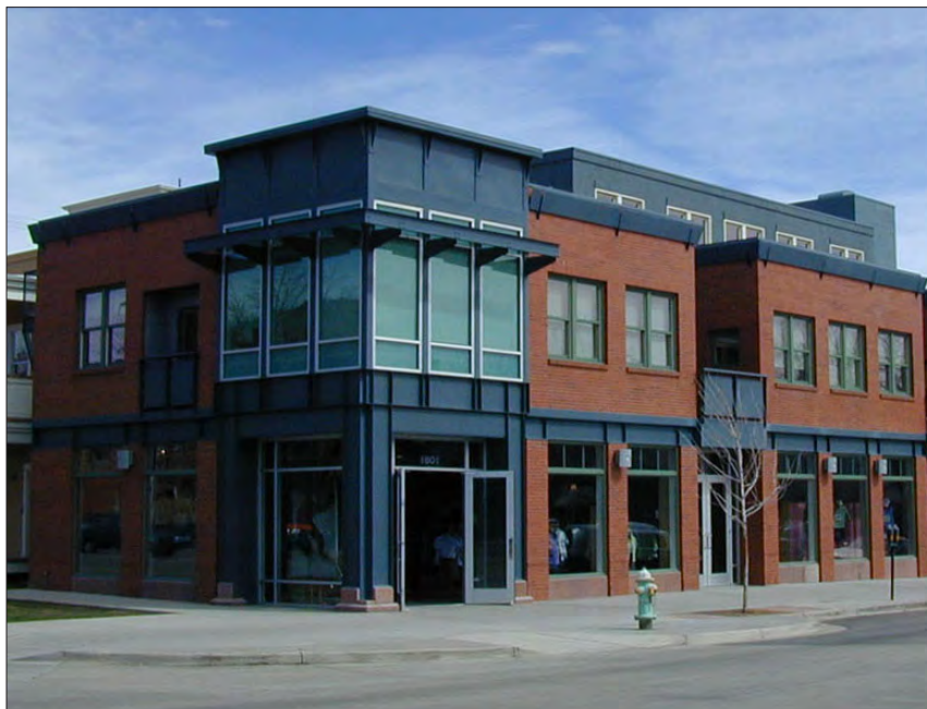
These buildings all incorporate the basic building blocks: (1) base, (2) middle and (3) cap. (Boulder, CO)
