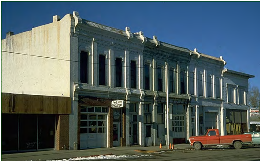
This row of buildings had lost some details over time. Overhead garage doors that had replaced original storefronts were later alterations without historic significance. Compare this photograph with the "after" photograph below. (Fort Collins, CO)
