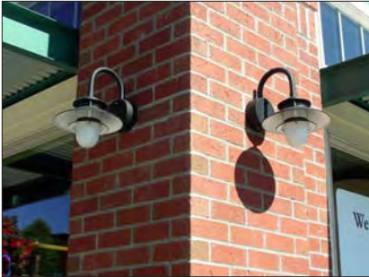
Use lighting fixtures that are appropriate to the building and its surroundings in terms of style, scale and intensity of illumination.
