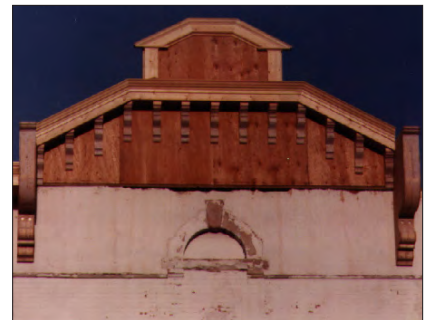
Reconstructing missing details using sufficient information is encouraged, this can be obtained from a historic photograph or investigation of physical evidence.
