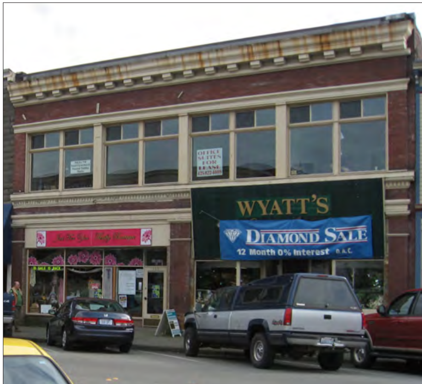
Italianate style commercial building on Main Street.
