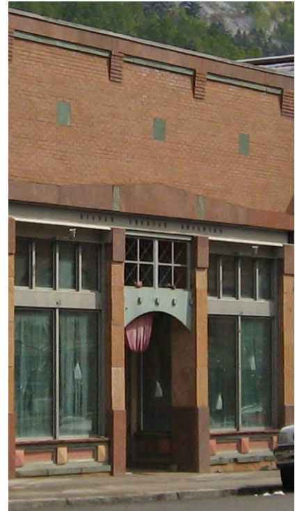
This contemporary interpretation of a storefront includes a recessed entry and transom element. (Telluride, CO)
