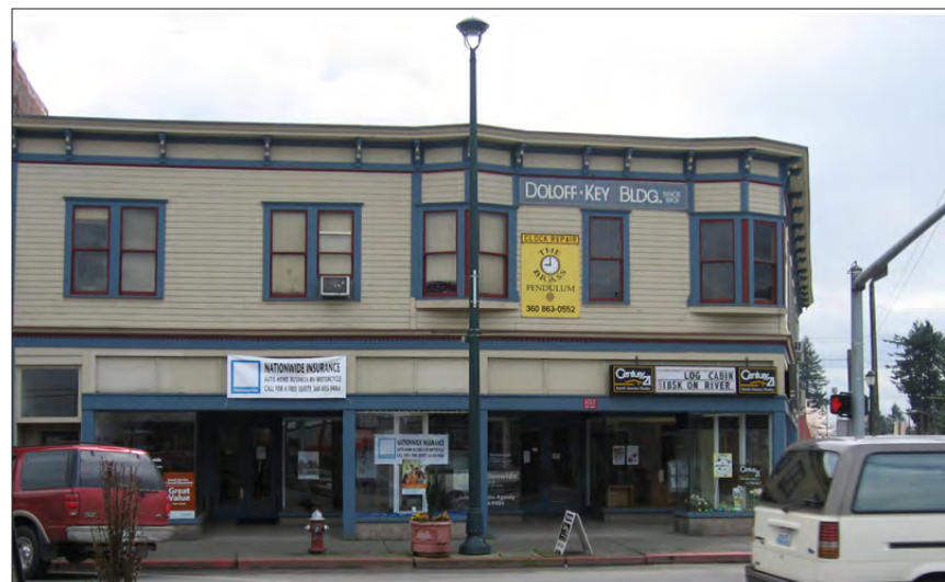
Preserve historic upper-story windows.
