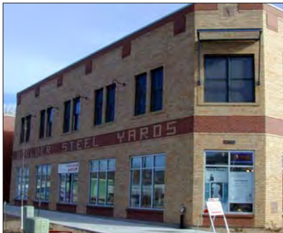
This building uses brick to delineate the base from the middle and a change in material color and architectural detailing to break down the apparent mass of the building. (Boulder, CO)
