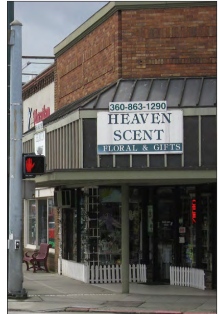
Consider restoring the historic storefront opening.
