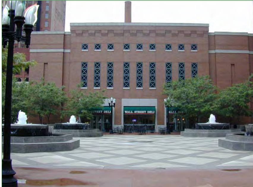
This parking structure has retail at the ground level and architectural ornamentation above to provide visual interest. (Louisville, KY)
