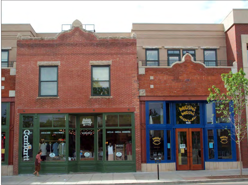
This third story addition is setback from the building front to maintain the traditional scale of the street facade. (Boulder, CO)
