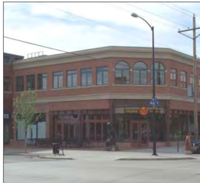
This building steps back on the corner which decreases the visual scale of the building. (Boulder, CO)
