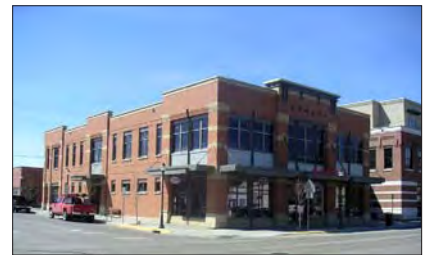
Divide larger building facades into "modules" that are similar in scale to buildings seen historically. (Bozeman, MT)
