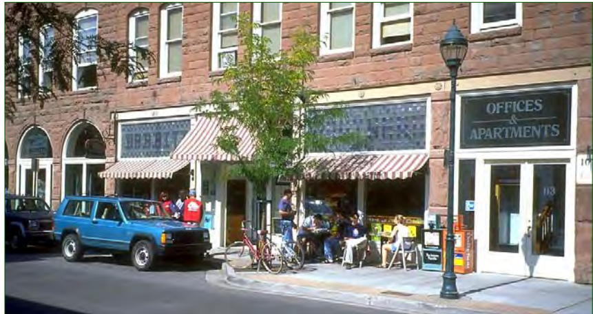
An appropriate dining area should be in front of the street wall. It is only appropriate to have outdoor dining when there is sufficient sidewalk width to allow for furniture and a comfortable walking path. (Flagstaff, AR)
