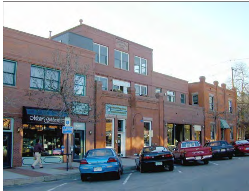
A roof addition should be set back from the primary, character-defining façade, to preserve the perception of the historic scale of the building. (Boulder, CO)
