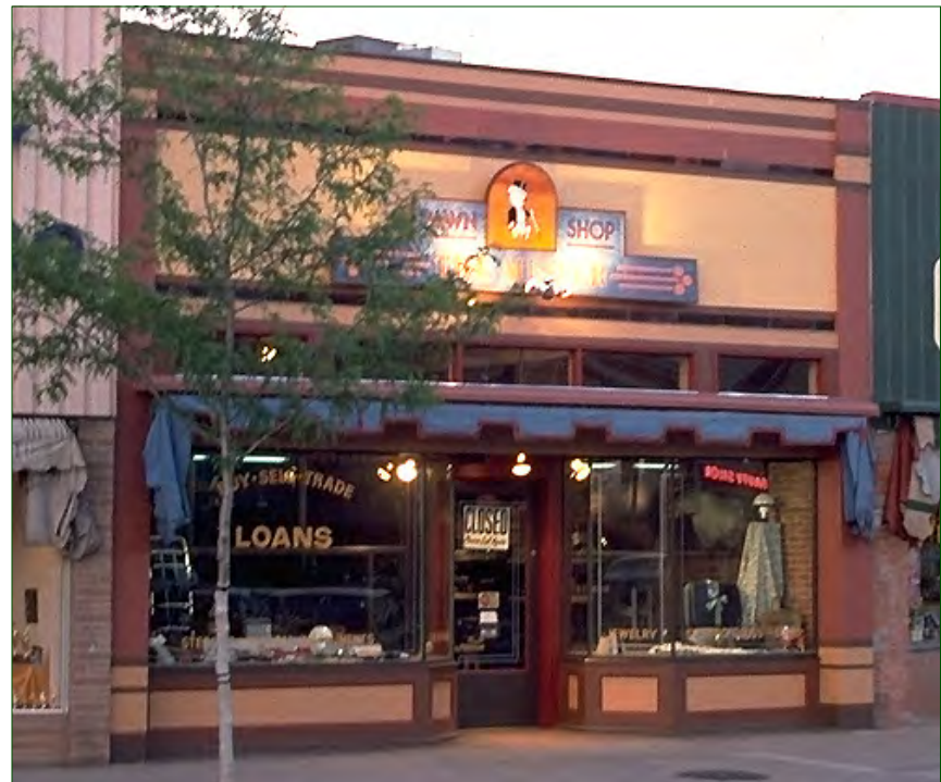
The same building (above) after renovation exhibits the more classical features of commercial storefronts, including a painted cornice, bulkhead and recessed entry. (Fort Collins, CO)
